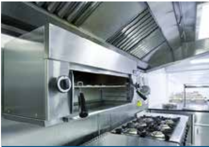
Kitchen Exhaust / Duct Maintenance
