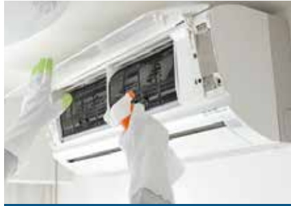
All Air Condition Maintenance
