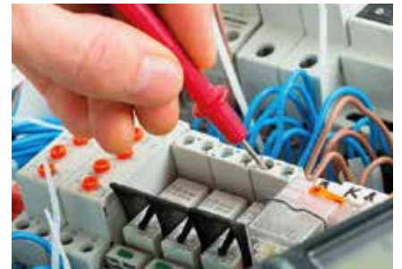
Electrical & Plumbing Work
